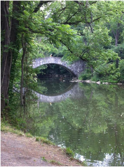
Anderson Stone Bridge
